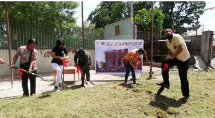
Groundbreaking for the construction of our “Alice Rose Clover Child Development Center”
